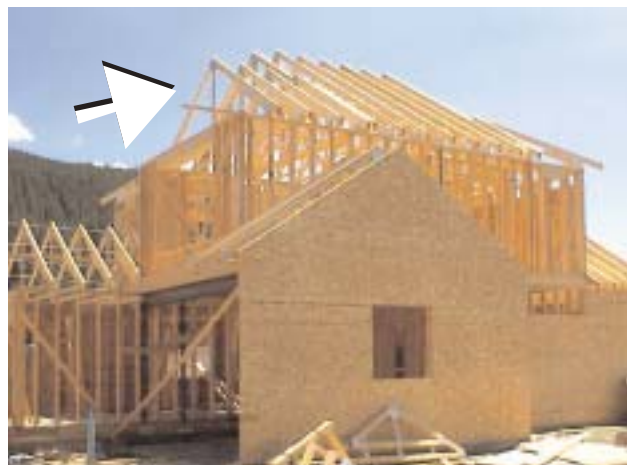
1-19 Pre-fabricated roof trusses in use
