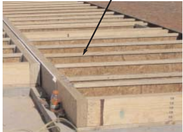
1-12 Framed wood floor system, using I-joists
