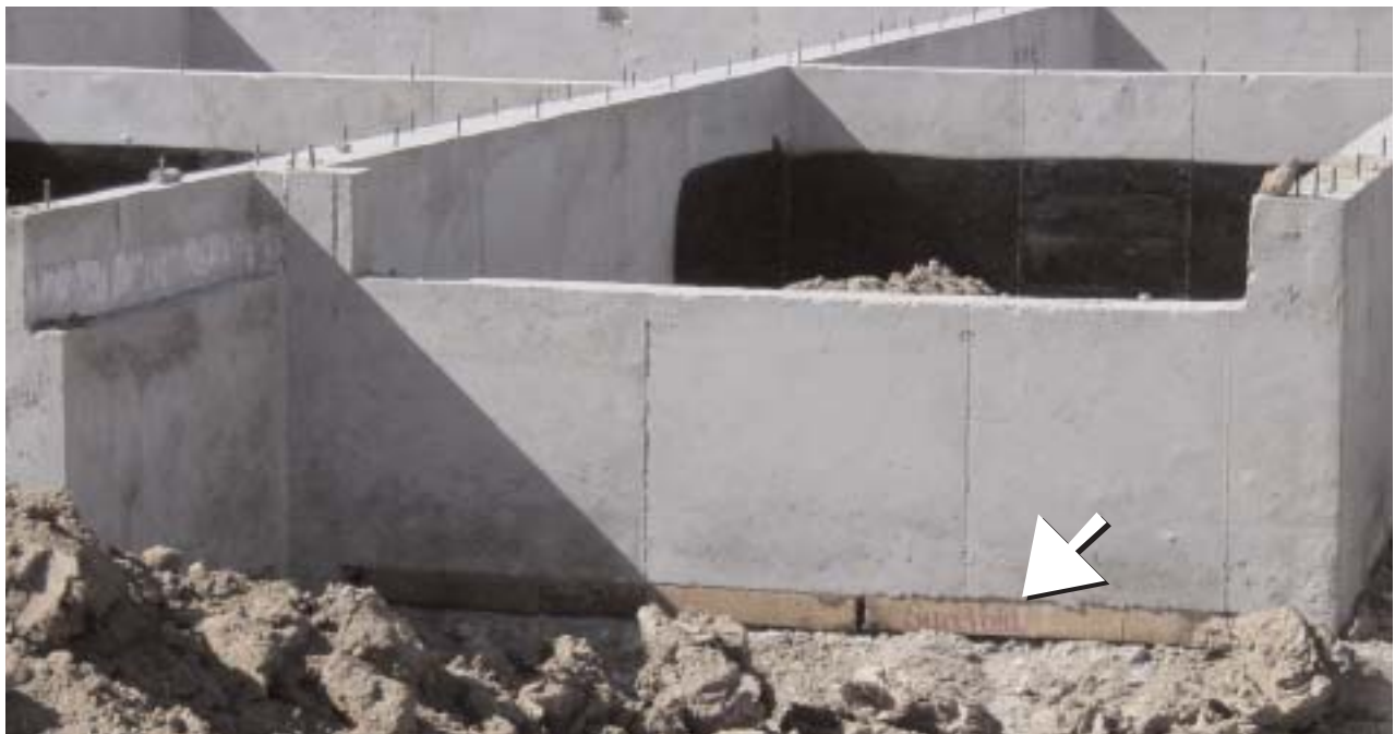
1-05 Compressible void material
