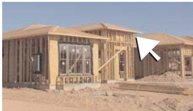
1-15 Bearing walls support the roof
