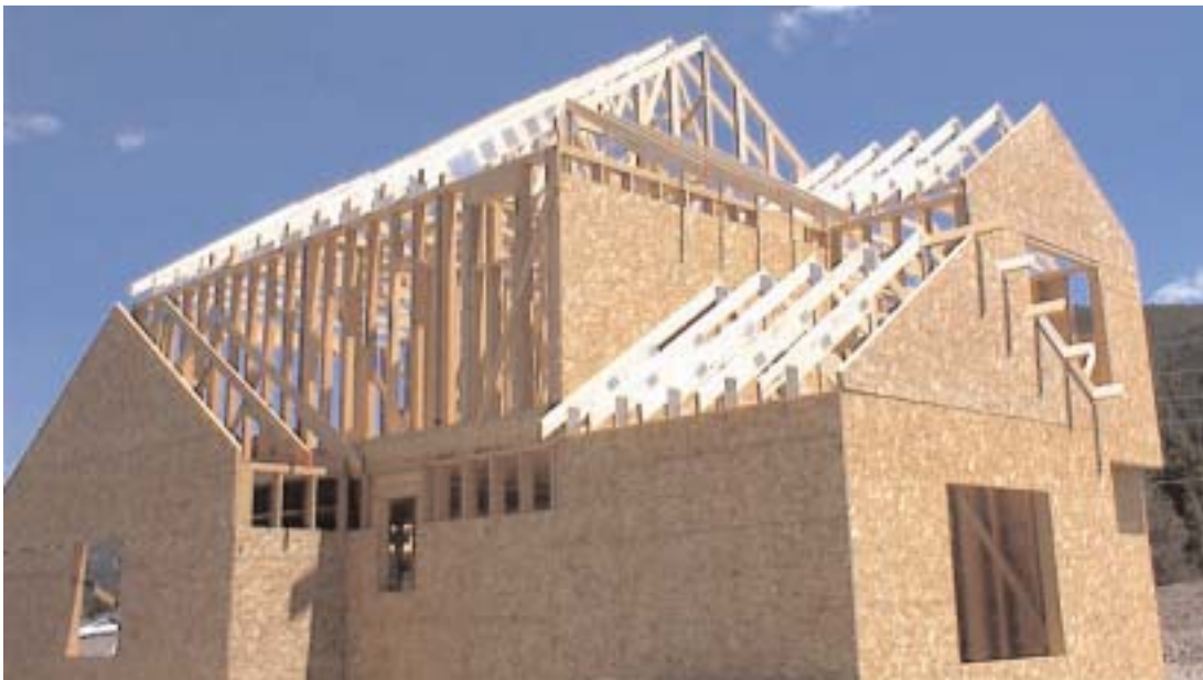
1-01 Load bearing walls supporting the roof
