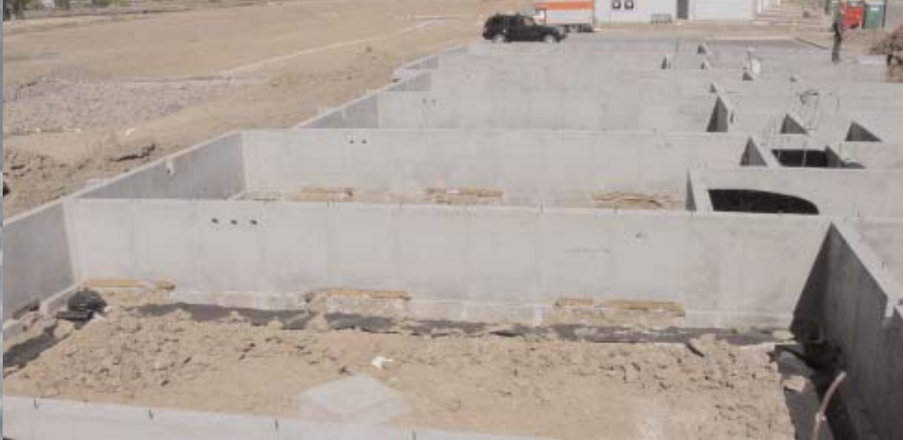
1-03 A grade beam on caisson foundation
