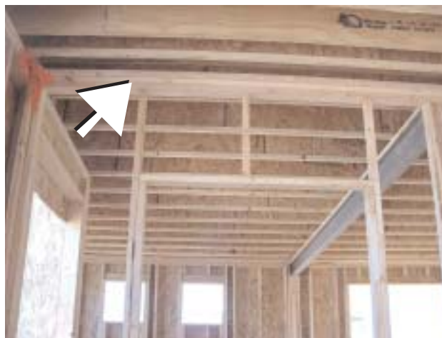
1-17 Non-load bearing wall (note that it does not support the ceiling)
