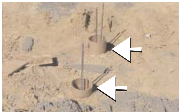
1-04 Caissons shortly after being poured
