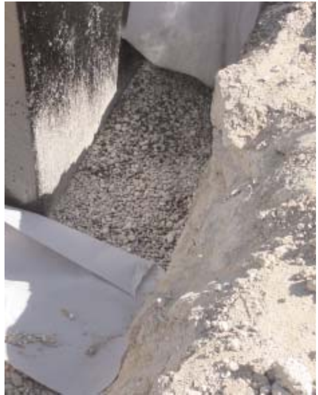
1-22 Foundation drain
