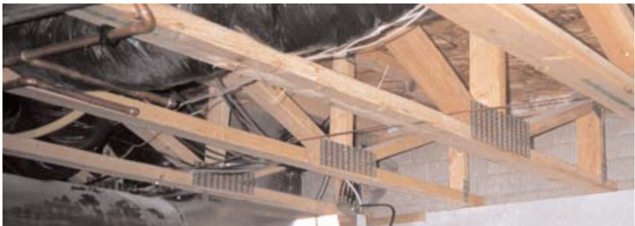
1-13 The underside of a floor built on fabricated floor trusses
