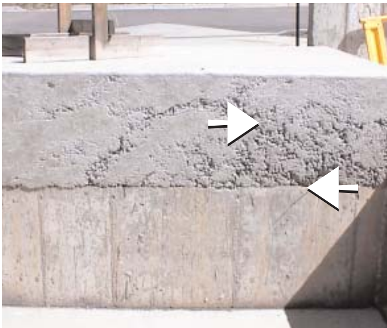
1-24 Cold joint (middle) with rock pockets (above)
