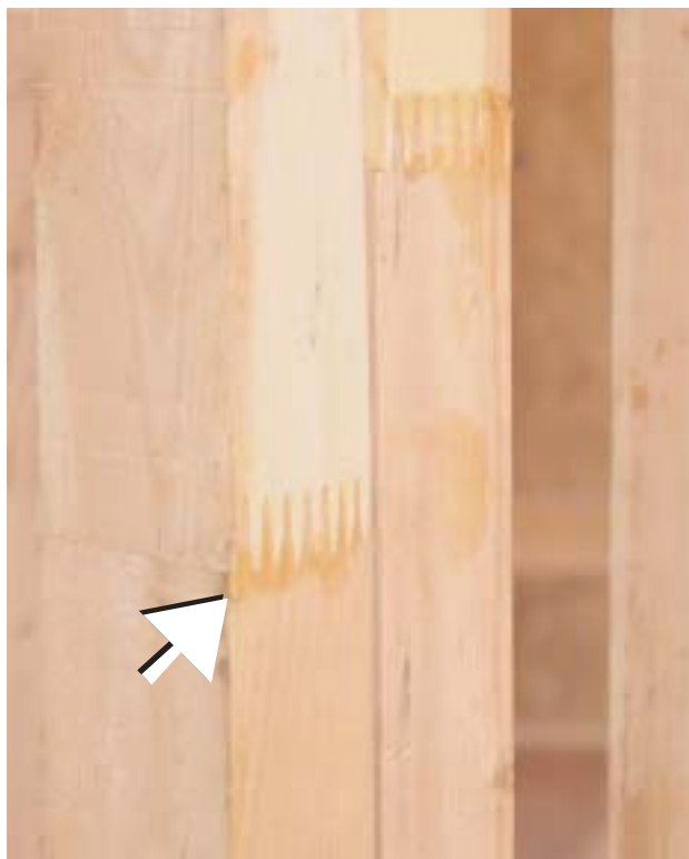
1-16 Finger jointed studs
