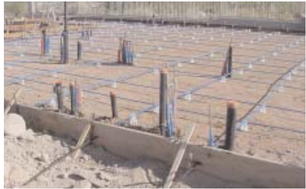
1-08 Form work set up for a poured-in-place foundation
