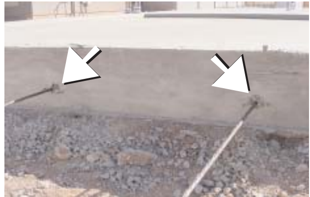
1-06 Slab on grade with tensioning cables
